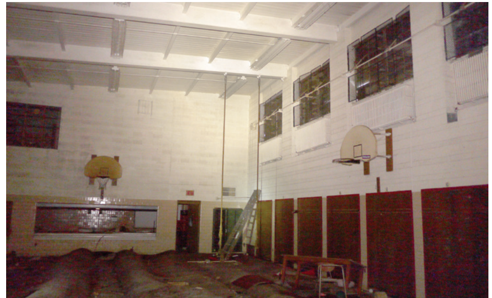
The gym doubled as a cafeteria, and includes an attached kitchen with wide serving window and dining tables that fold out from the walls. A row of high steel-frame clerestory windows provide natural light.
