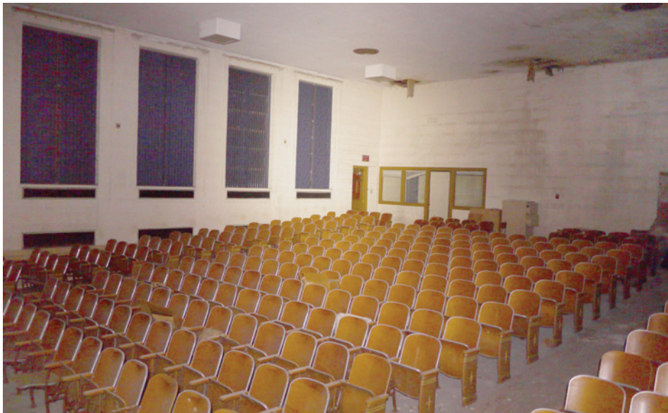
The auditorium, added in 1952, is a simple CMU box. Original wood seating and steel-frame windows are still intact.
