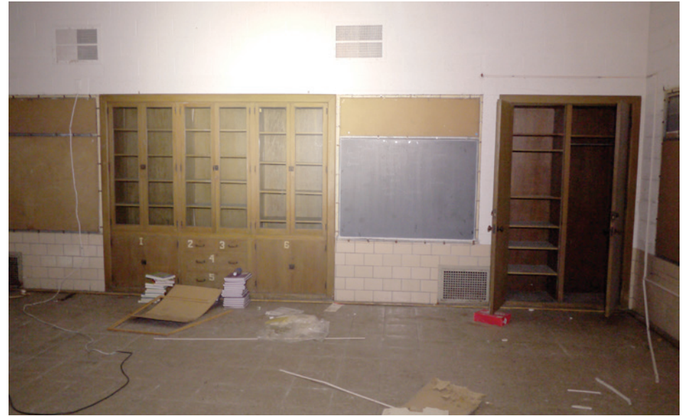
Classrooms feature simple and durable finishes: CMU walls, acoustic tile ceilings, VCT floors, and simple wood cabinetry.
