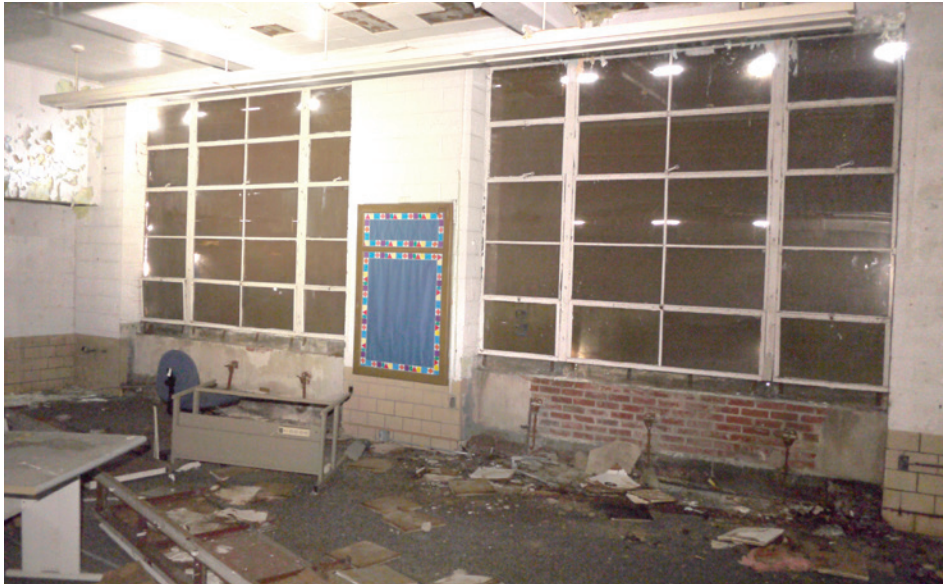
Classrooms feature large double windows consisting of a 4x5 steel-frame grid. Most of the original windows at Parkman remain intact.
