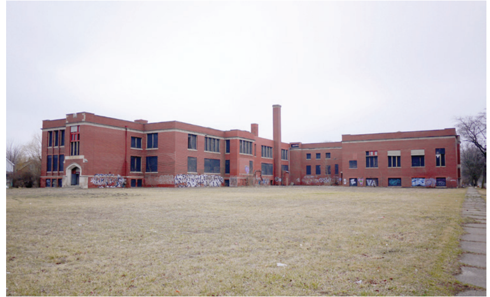
Rear elevations and spacious school yard viewed from the northwest. The school is one of the largest elementary schools included in this study.
