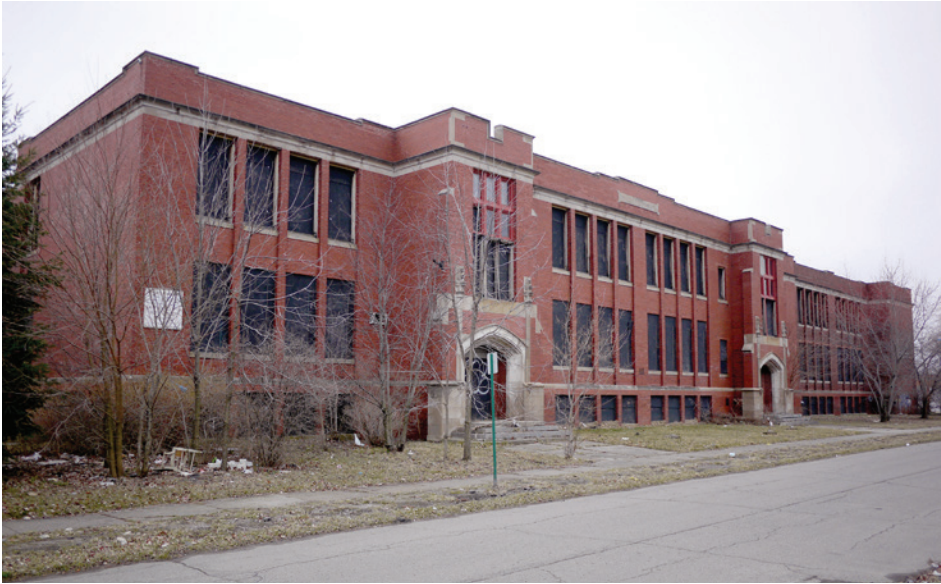
The original 1912 building's front elevation featured a symmetrical design anchored by two large entry towers. The 1922 classroom extension is visible in the background.
