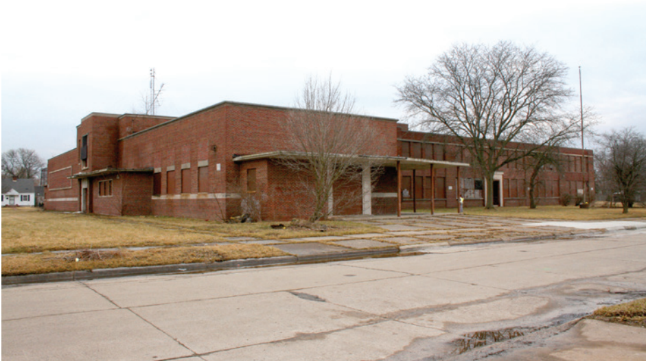
Exterior viewed from the northwest corner. The 1951 auditorium is visible in the foreground, with the gym located behind (far left of frame). The original 1920s classroom wing is visible on the right.
