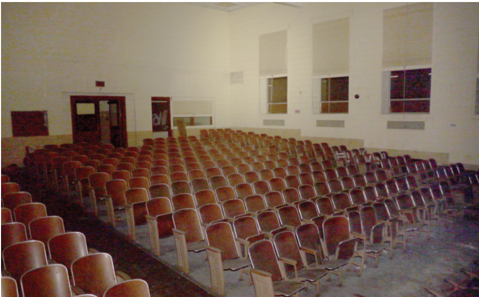
The auditorium is utilitarian CMU construction with no frills. While it is not a particularly beautiful or impressive space, it is solidly built and in relatively good condition. There is a dedicated entrance with vestibule and covered sidewalk near the street.
