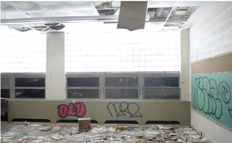
A typical classroom in the 1951 wing, featuring large glass block windows with operable steel frame lites below. The more durable painted CMU finishes in the newer wing are in relatively good shape compared to the moisture-sensitive plaster of the 1920s wing.
